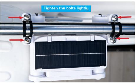
Use the smallest possible metal clamp. If the originally installed metal clamp is too small, you can replace it with a 16mm metal clamp (provided). It is best to use the **smallest** possible metal clamp.
